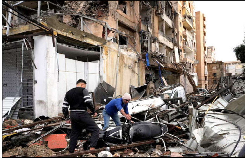
A man moves a scooter amid the rubble, in the aftermath of Israeli strikes on Beirut's southern suburbs, amid the ongoing hostilities between Hezbollah and Israeli forces, in Lebanon.
