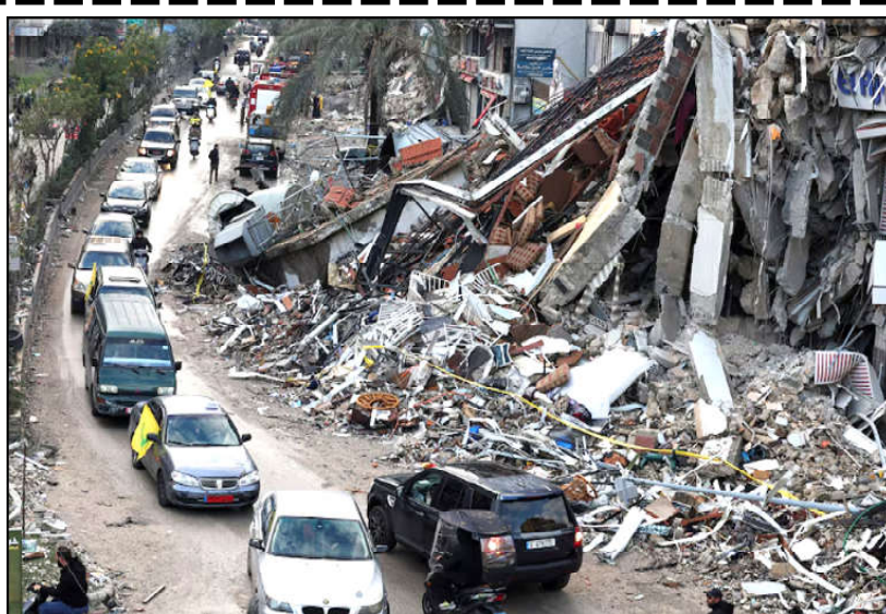
Vehicles drive near damaged buildings in Beirut's southern suburbs, after a ceasefire between Israel and Hezbollah took effect, in Lebanon.
