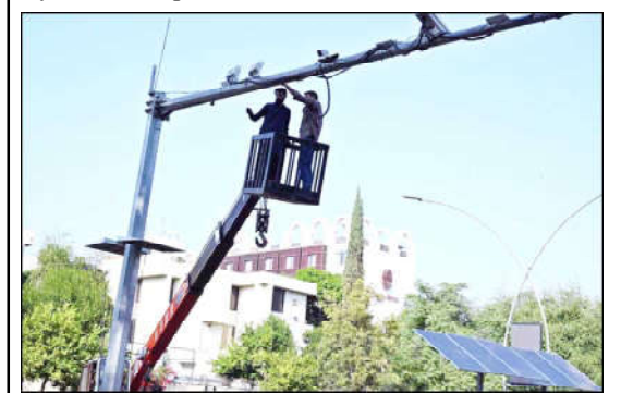
ISLAMABAD: Worker busy repairing security cameras in Federal Capital.
