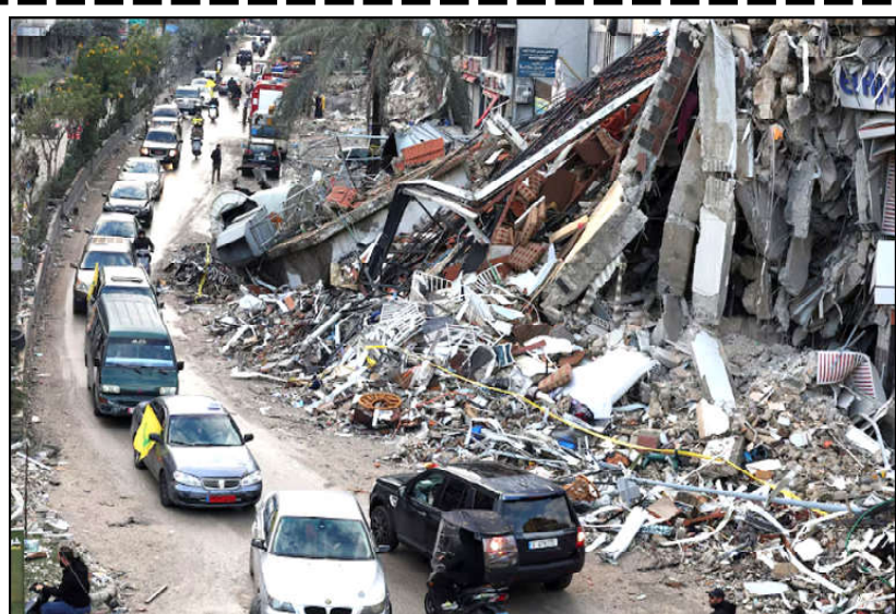
Vehicles drive near damaged buildings in Beirut's southern suburbs, after a ceasefire between Israel and Hezbollah took effect, in Lebanon.
