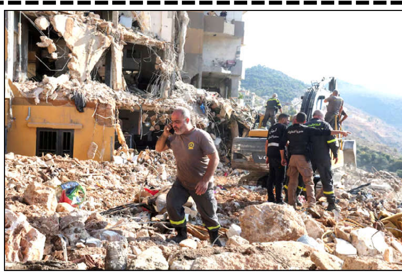
Civil defense members work at a site damaged in the aftermath of an Israeli strike, amid the ongoing hostilities between Hezbollah and Israeli forces, in Barja, Lebanon.
