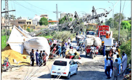
HYDERABAD: An electric pole has fallen due to a truck collision at Tando Yousuf Road.
