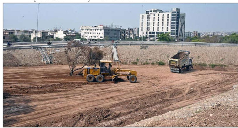
ISLAMABAD: Machinery is being used for leveling the ground to prepare a green area along the road near Kakpul.
