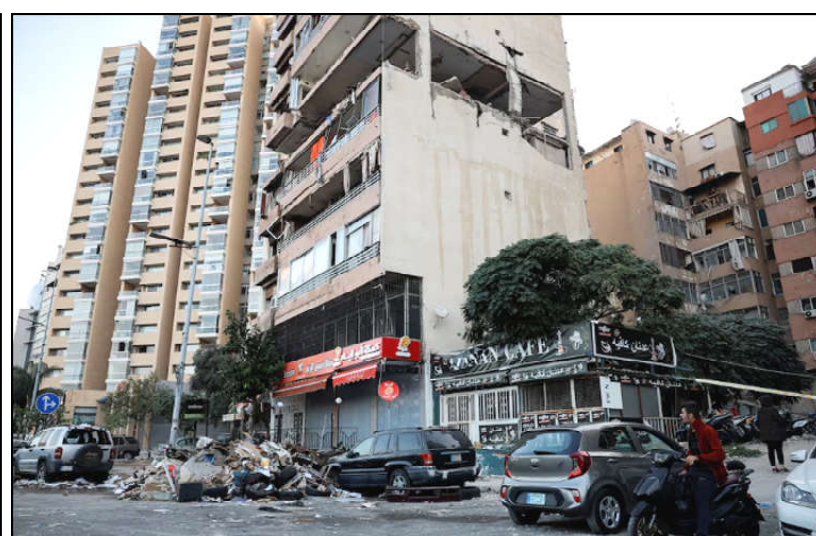
People pass by buildings damaged in an Israeli strike, amid ongoing cross-border hostilities between Hezbollah and Israeli forces, in Kola, central Beirut, Lebanon.
