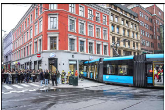
A crowd gathers to watch as first responders work after a tram derailed and crashed into a building in the center of Oslo, Norway.
