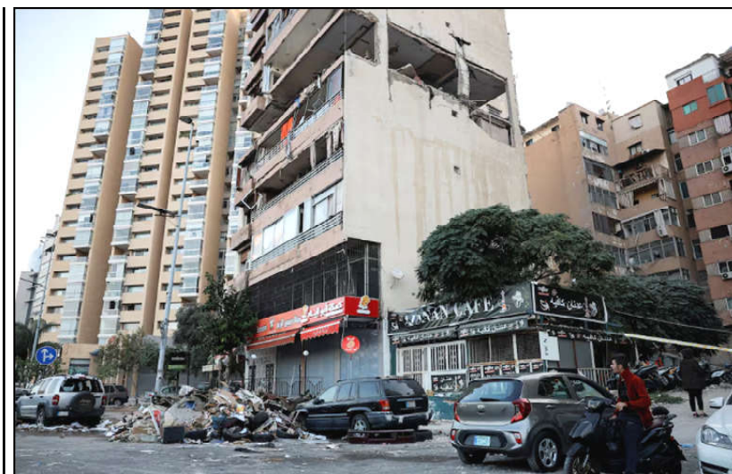
People pass by buildings damaged in an Israeli strike, amid ongoing cross-border hostilities between Hezbollah and Israeli forces, in Kola, central Beirut, Lebanon.
