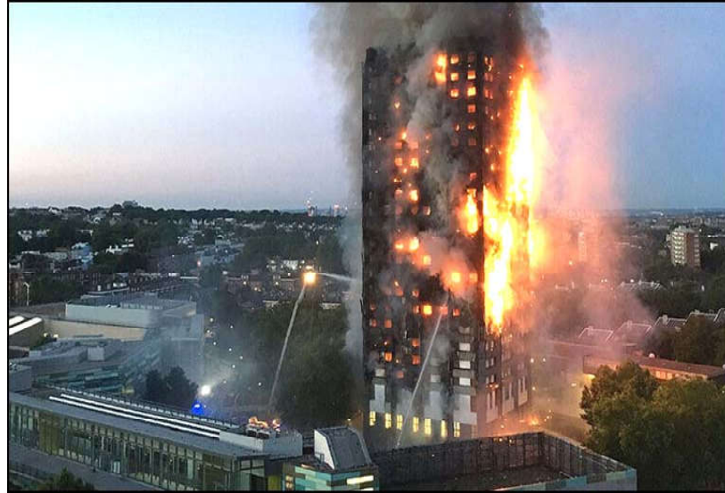
Flames and smoke coming from a 27-storey block of flats after a fire broke out in west London.
