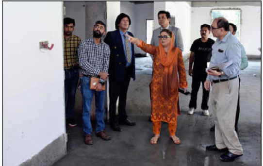
LAHORE: Punjab Information Minister Azma Bukhari inspecting the newly constructed building of DGPR, Punjab Secretary Information and DGPR Shenshah Faisal Azeem is also present.
