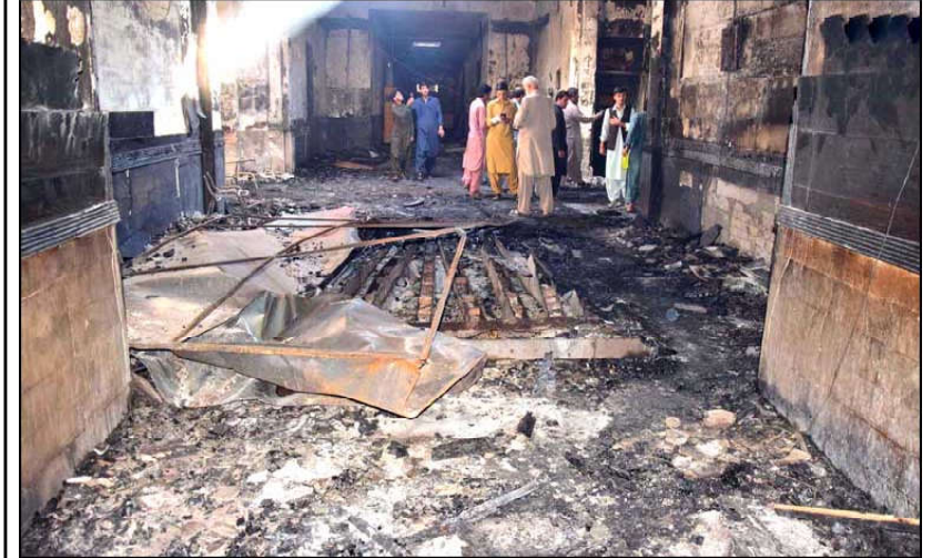
QUETTA: A view of damages due to fire at Science College
