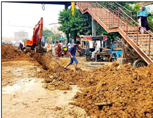
KARACHI: Labourers busy in digging for laying pipeline at Liaquatabad area.
