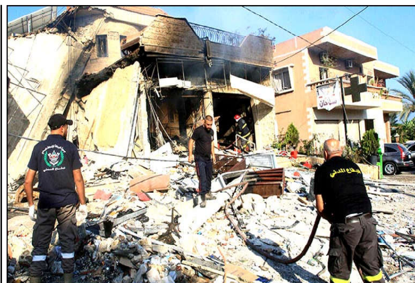
Rescuers inspect the debris at the site of an overnight Israeli strike on a pharmacy in the southern Lebanese village of Akbiyeh.
