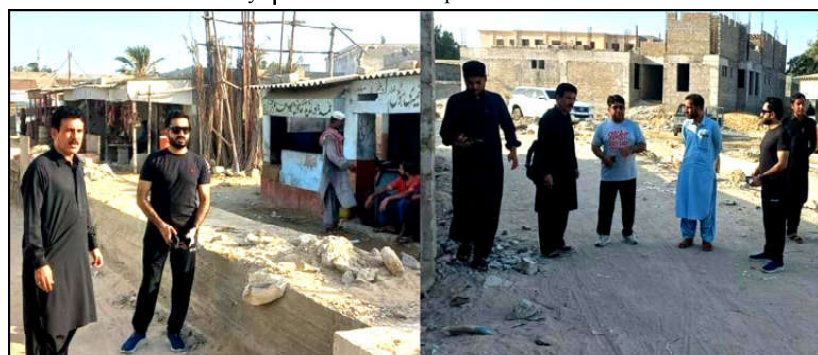
GWADAR: Director General GDA Shafqat Anwar Shahwani alongwith Assistant Commissioner Mir Jawad Ahmed Zehri inspecting under construction sewerage line project under Master Plan
