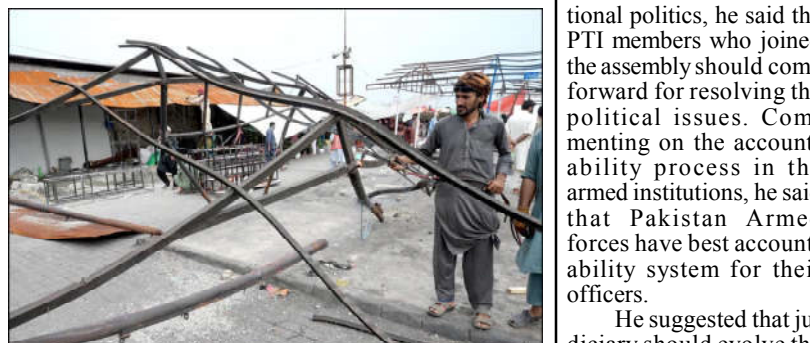
ISLAMABAD: CDA workers work on restoring stalls after the fire at H-9 weekly bazaar in the Federal Capital
