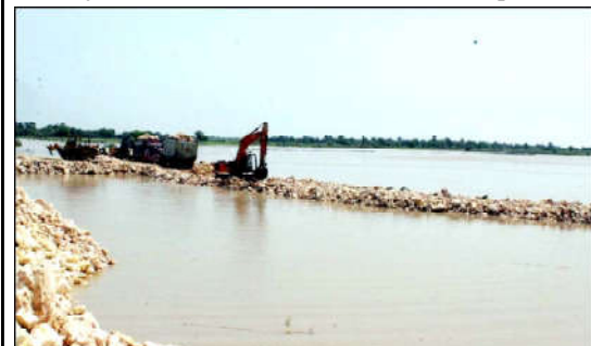
LARKANA: Moria Loop Bund is being strengthening by the bank of River Indus, in perception of arrival of flood water in the Indus Rive, pressure of water increased day by day on the embankment, near Larkana.
