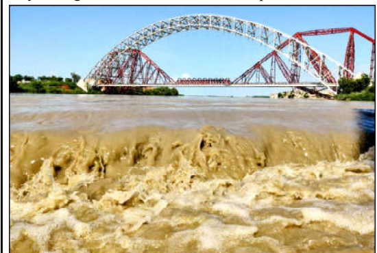
SUKKUR: Water level increases while medium grade flood water reaches at Sukkur Barrage on River Indus due to heavy downpour of monsoon season, in Sukkur.
