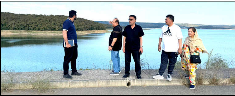
ISTANBUL: Balochistan Minister for Irrigation Mir Muhammad Sadiq Umrani visiting Omerli Dam in District Çekmeköy
