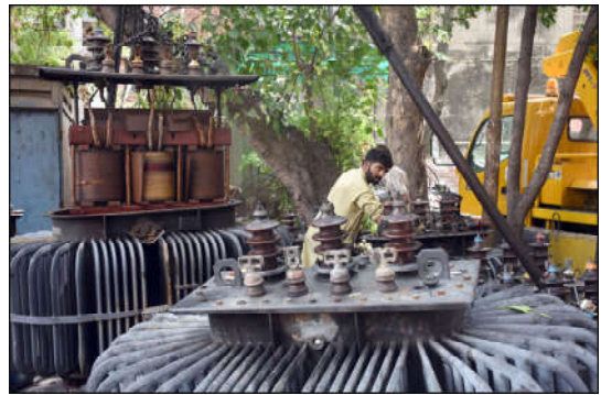
LAHORE: AWAPDA engineer is busy in repairing Transformers at G.R.O in the Federal Capital
