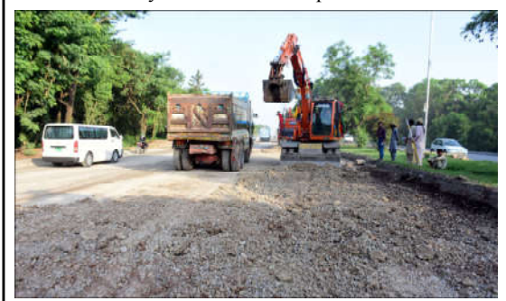
ISLAMABAD: Work in progress on Park Road expansion project in the Federal Capital.
