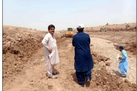
NASEERABAD: Heavy machineries busy in cleaning and maintenance Rabi Canal during cleanliness drive under the supervision of Irrigation Department, in Naseerabad.
