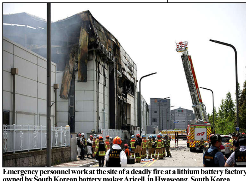
Emergency personnel work at the site of a deadly fire at a lithium battery factory owned by South Korean battery maker Aricell, in Hwaseong, South Korea.
