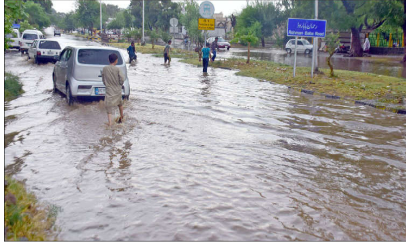
ISLAMABAD: After heavy rain and hail in the federal capital, the roads are looking like ponds. A serious problem of water drainage, the rains controverts the CDA's tall claims.
