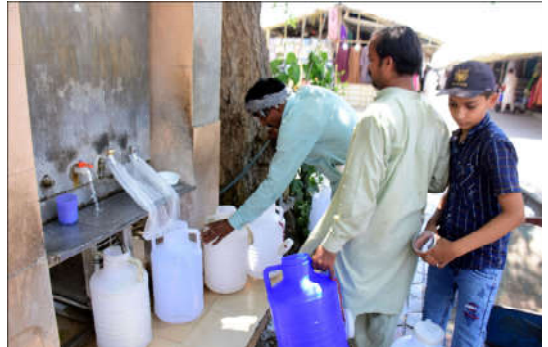
ISLAMABAD: People taking drinking water at a filtration plant installed at Sector II-9 in the Federal Capital.
