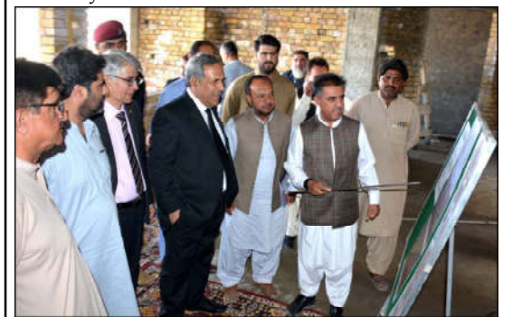
QUETTA: Chief Justice Balochistan High Court, Mr. Justice Hashim Khan Kakar being briefed about newly constructed building of Balochistan Civil Services Academy.
