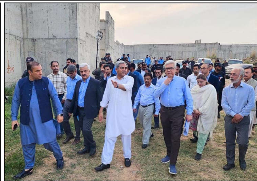
ISLAMABAD: Federal Minister for Interior Mohsin Naqvi visiting the under construction Model Prison.
