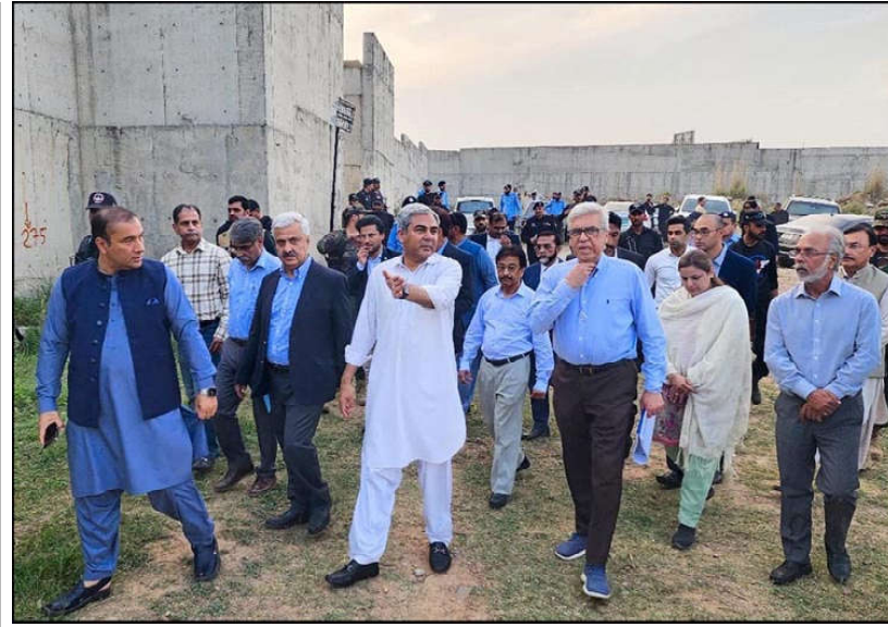
ISLAMABAD: Federal Minister for Interior Mohsin Naqvi visiting the under construction Model Prison.
