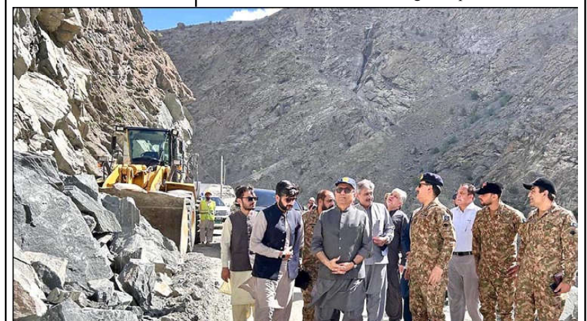
SKARDU: Federal Minister for Communications, Privatization & Board of Investment, Abdul Aleem Khan inspecting land slide in Skardu.
