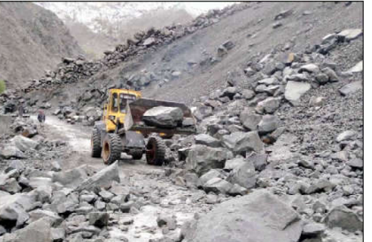
GILGIT: Workers of Gilgit-Baltistan Disaster Management Authority and GBPWD busy in clearing blocked road of Astore after heavy rain and land sliding in the area.
