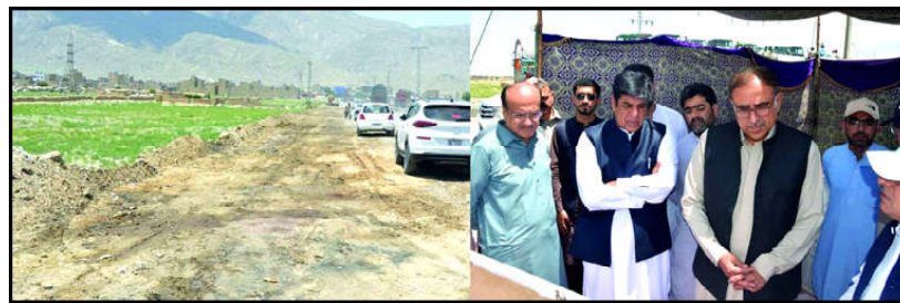
QUETTA: Provincial Minister for Communication & Works Mir Saleem Ahmed Khosa and Secretary C&W Qambar Dashti being briefed about expansion of Gai Khan Chowk to Western bypass road.
