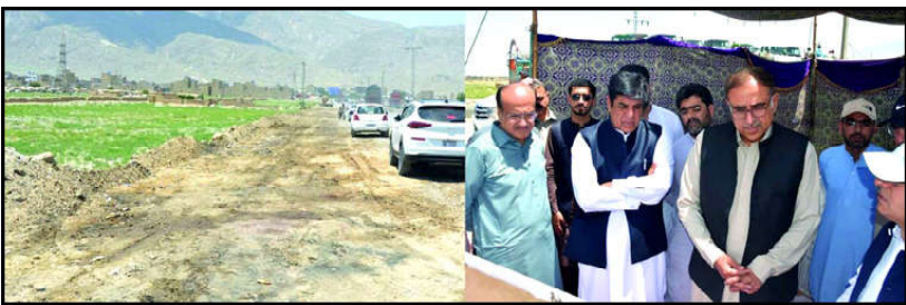
QUETTA: Provincial Minister for Communication & Works Mir Saleem Ahmed Khosa and Secretary C&W Qambar Dashti being briefed about expansion of Gai Khan Chowk to Western bypass road.
