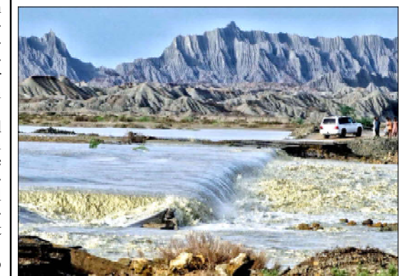
HUB: View of Pishukan to Gwadar link Shabi bridge once again washed away in water relay after massive rainfall in Hub
