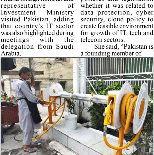
SIALKOT: A person filling water in pot at water filtration plant with petrol pump style water nozzle at Mubarak Pura.
