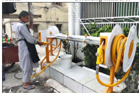
SIALKOT: A person filling water in pot at water filtration plant with petrol pump style water nozzle at Mubarak Pura.
