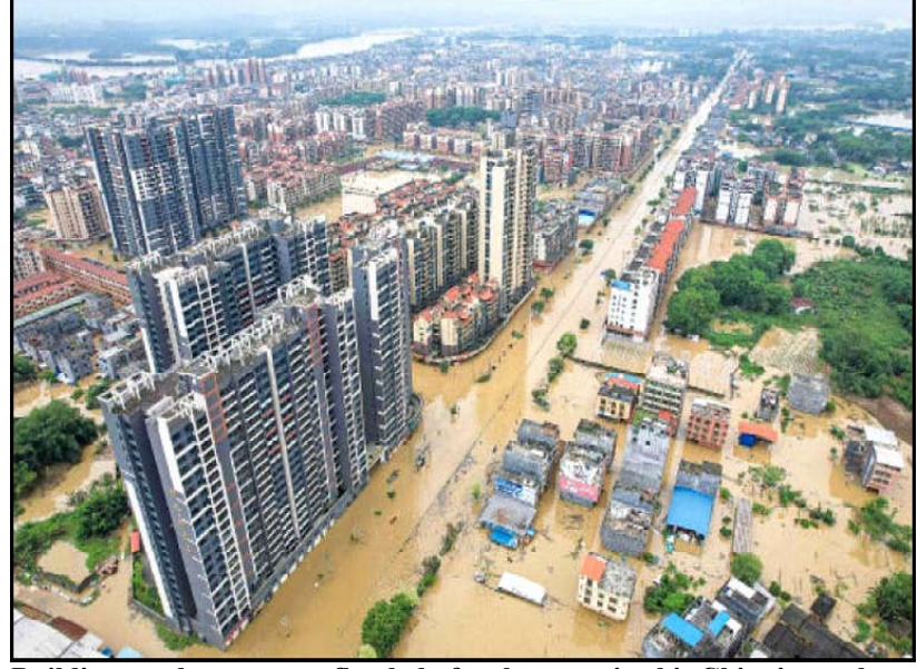
Buildings and streets are flooded after heavy rains hit China's southern Guangdong province.
