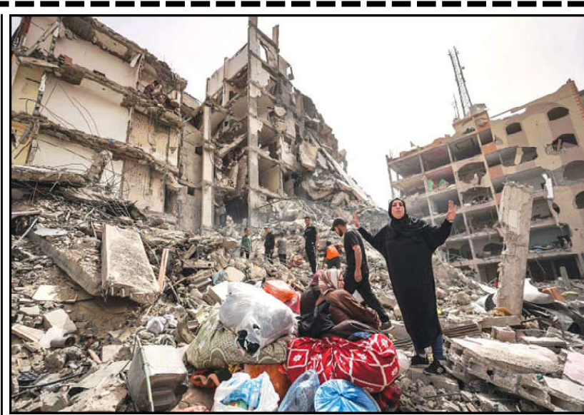
Palestinians attempt to salvage their belongings from the rubble of a damaged building in the city of Nuseirat, in central Gaza Strip.
