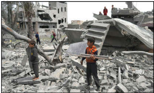
Palestinians inspect the damage to a building, following Israeli bombardment, in the Maghazi camp for Palestinian refugees in the central Gaza Strip.
