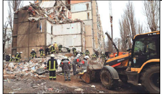
Rescuers work at the site of a heavily damaged apartment building in Odesa, following a Russian drone attack.
