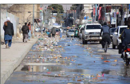
QUETTA: A view of accumulated sewerage water on imdad chowk crating problems for locals.
