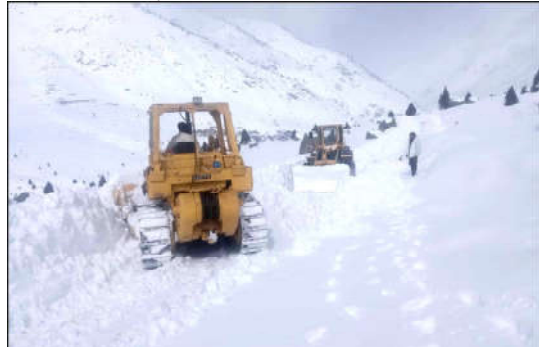
ASTORE: Heavy machinery being used to remove snow and boulders from the blocked road of Astore Valley by the staffer of Gilgit-Baltistan Disaster Management authority and Works Department after heavy snow fall and rain in area caused land sliding in diffident area.
