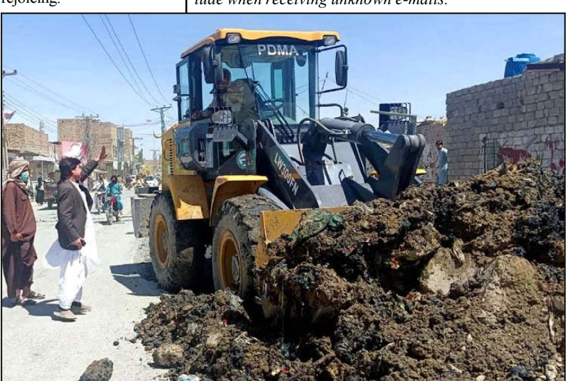
QUETTA: Workers are busy in cleaning works of sewerage drain over the directions of Metropolitan Corporation Administrator Hamza Shafaqat.
