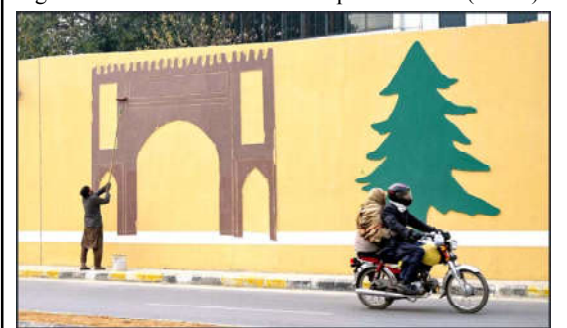
ISLAMABAD: A skilled person paints the wall of 7th Avenue underpass near Aabpara Market.
