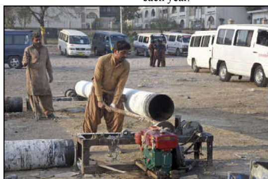
ISLAMABAD: Labourers are busy installing new water pipeline at sector F-5 in the Federal Capital.
