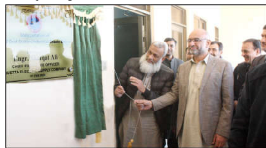
QUETTA: Chief Executive Officer QESCO Engr. Shafqat Ali inaugurating newly constructed 132 KV Industrial Estate Bostan Grid Station
