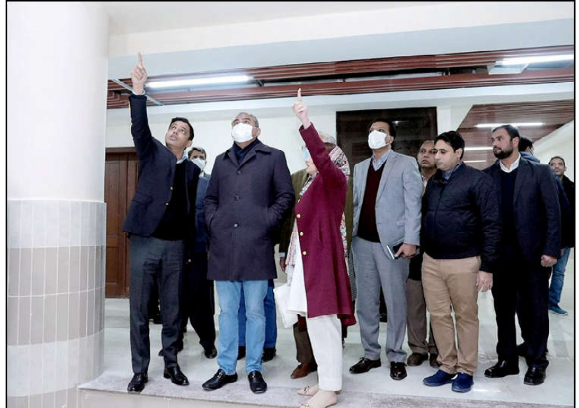
LAHORE: Caretaker Chief Minister Punjab Mohsin Naqvi inspecting under Construction Works at Fatima Jinnah Institute of Dental Sciences at Jubilee Town.
