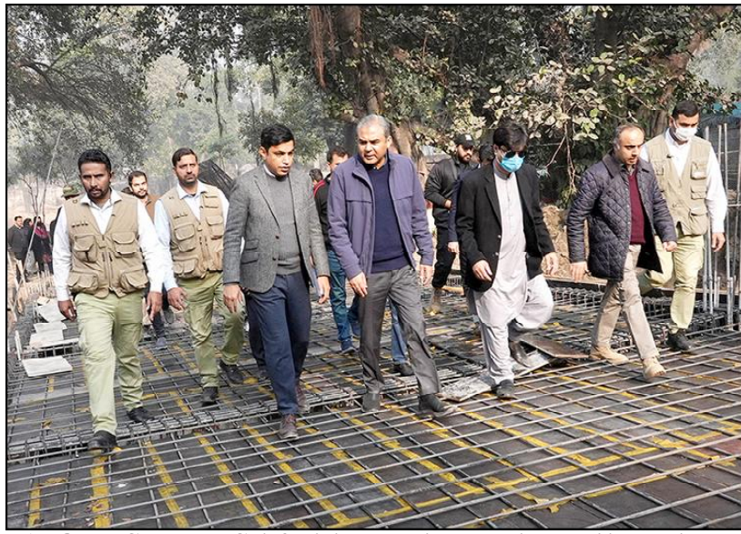
LAHORE: Caretaker Chief Minister Punjab Mohsin Naqvi inspecting the on-going construction works at Lahore Zoo.
