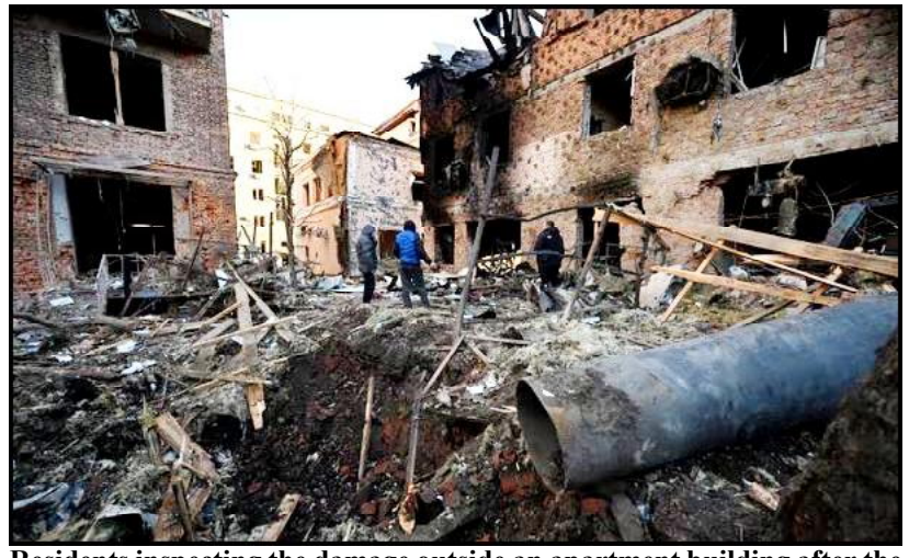
Residents inspecting the damage outside an apartment building after the overnight Russian drone attack in Kharkiv.
