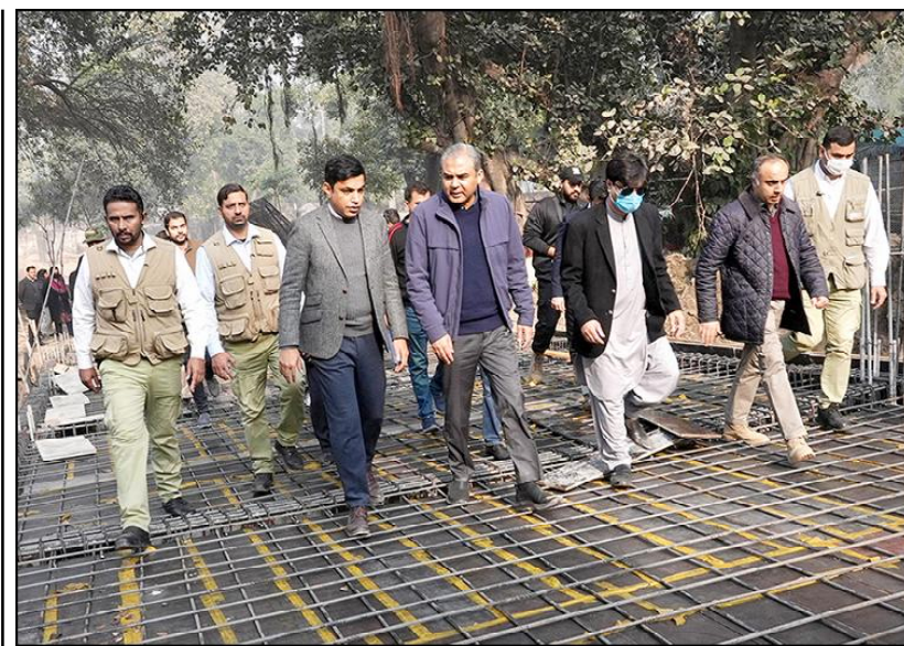
LAHORE: Caretaker Chief Minister Punjab Mohsin Naqvi inspecting the on-going construction works at Lahore Zoo.
